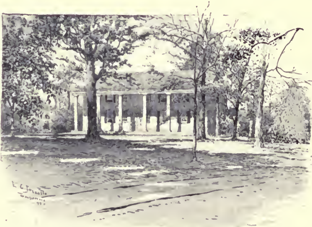
THE HOME OF GENERAL PHILIP SCHUYLER AT OLD SARATOGA, NEAR SCHUYLERVILLE.
